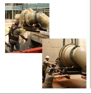
Hunton Services replaced all 5 of the chillers that were original equipment when the property was first built in 1982: 3 - 1,400-ton units, an 800-ton unit and a 400-ton unit. Also replaced were 2 exhaust fans that comprise a ventilation portal, a refrigeration monitor that tracks HVAC system leakage as well as numerous valves and actuators that were critical to achieving the property's LEED Gold energy-efficiency certification.
