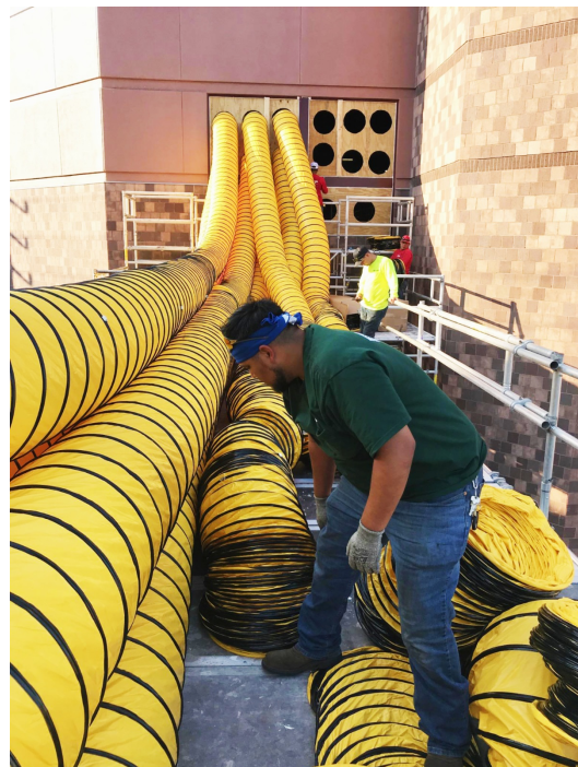
Hunton Rental Solutions Technician Setting up Duct
